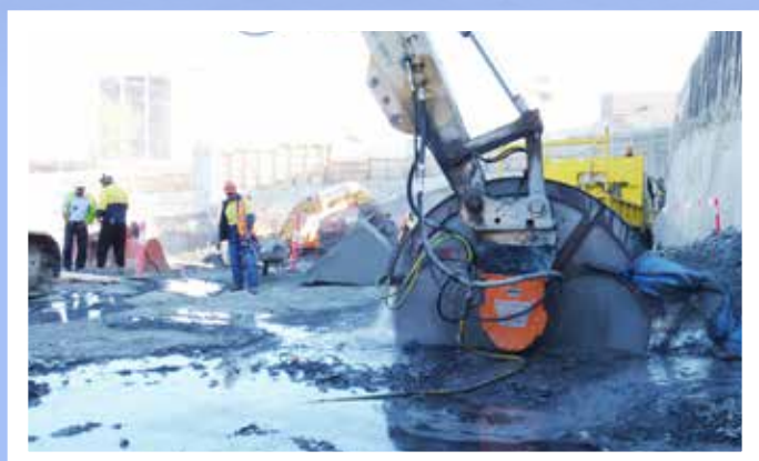
📍 Echidna D6 diamond rocksaw with 2500mm blade cutting hard sandstone for a shopping centre carpark. (Wollongong, Australia)
