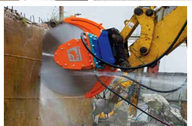
📍 High speed D4HS diamond rocksaw used for demolition of hard, reinforced concrete. (Czech Republic)
