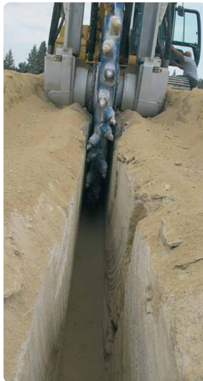
ERW 1000 trenching in medium hard limestone
