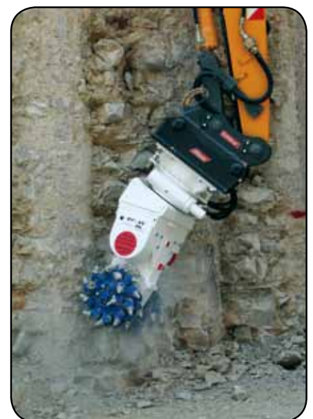
Used in foundation application
