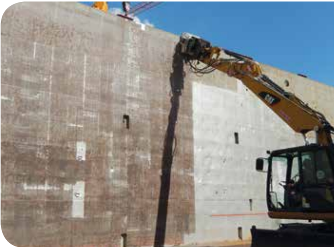
Excavator attachment for the cleaning of metallic surfaces Hearing protection must be worn while working with the EXRUST cleaning heads.
