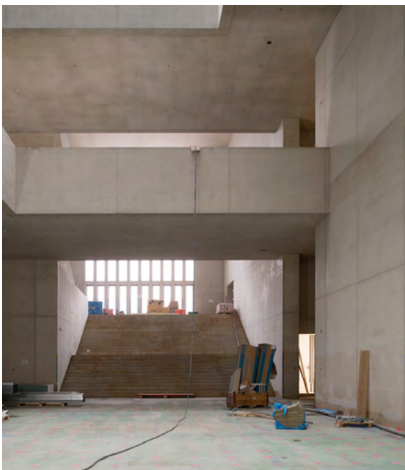
Recycled concrete in the new Kunstmuseum building in Zurich
